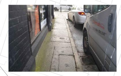
REVIEW MINIMUM WIDTH OF FOOTPATH: -1500MM. WHEN OBSTACLES CANNOT BE REMOVED AND 1200MM. IN A DISTANCE OF 2000MM.
