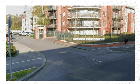
UNCONTROLLED CROSSING OF A SHARED ROUTE! CORDUROY TACTILE SURFACE SHOULD BE INSTALLED FOR A DEPTH OF 2400MM ON EITHER SIDE OF THE JUNCTION. FOR PEDESTRIANS (PERPENDICULAR) AND CYCLISTS (PARALLEL), TO INDICATE THE START/END OF THE ROUTE. A BLISTER SURFACE OF 1200 mm DEPTH. SHOULD BE LAID ACROSS THE FULL WIDTH OF THE CROSSING POINT
