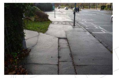
UNEVEN SURFACES IN THE FOOTPATH SHOULD BE CHECKED AND VERTICAL DEVIATIONS OF MORE THAN 5MM. IN CONCRETE SLABS TO BE AVOIDED.
