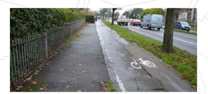
CRACKED PAVEMENT IN THE SHARED ROUTE. NO VISUAL DISTINCTION BETWEEN PEDESTRUAN AND CYCLIST PATH. PAVEMENT SHOULD BE REPAIRED WITH A PROPER PAINT MARKS.
