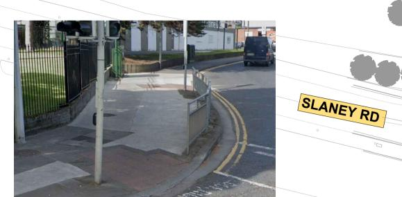
THE STEMS OF THE CONTROLLED CROSSING SHOULD EXTEND TO THE REAR OF THE FOOTPATH FOR THE CORRECT ORIENTATION OF PEOPLE WITH VISUAL IMPAIRMENTS
