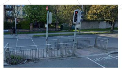
STAGGERED CROSSING POINTS IN THE DESIGN PROJECT TO BE REVIEWED. A CENTRAL REFUGE ISLAND IN ONE STAGE WITH PROPER RED BLISTER TACTILE PAVING SHOULD BE RECOMMENDED TO AVOID PEOPLE TO GET STUCK BECAUSE OF THE NARROW WIDTH.
