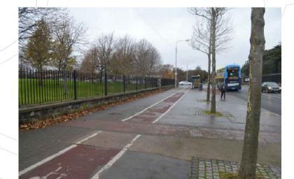
ADEQUATE TACTILE PAVING SURFACE (CORDUROY) SHOULD BE PROVIDED BEFORE THE INTERSECTION WITH THE STEM OF THE CONTROLLED CROSSING, IN THE CYCLE TRACK AND IN THE FOOTPATH.
