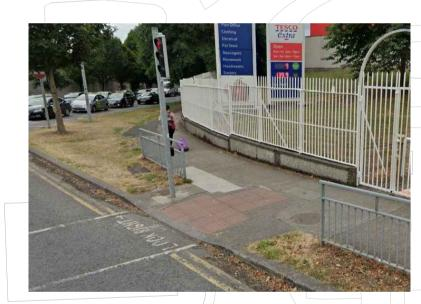
THE STEM OF TACTILE PAVING SURFACE IN THE CONTROLLED CROSSING POINT SHOULD EXTEND TO THE REAR OF FOOTPATH. AT THE CROSSING POINT. THE TACTILE PAVING SHOULD BE LAID ACROSS THE FULL WIDTH OF THE DROPPED KERB. THIS SHOULD BE A MINIMUM OF 2.4M WIDE AND SHOULD BE 800MM (2 SLABS) DEEP. THE TOP OF THE DROPPED KERB AT THE CROSSING SHOULD BE PAINTED WHITE FOR THE BENEFIT OF PARTIALLY SIGHTED PEDESTRIANS. AUDIBLE "BLEEP AND SWEEP" AND TACTILE DEVICES SHOULD BE IMPLEMENTED.
