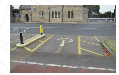
ABSENCE OF DISHED KERB FOR DISABLED PEOPLE. A DISHED KERB SHOULD BE PROVIDED WITH A SLIP-RESISTANT SURFACE AND A MINIMUM WIDTH OF 1200MM AND MINIMUM GRADIENT OF 1:12. THE ACCESSIBLE PARKING SPACE SHOULD BE ON FIRM AND LEVEL GROUND WITH NO VARIATION OF SURFACE EXCEEDING 5 MM.
