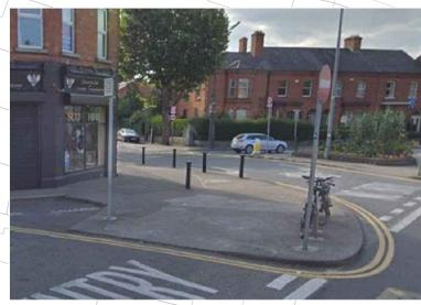
UNCONTROLLED CROSSING POINT. NO DISHED KERBS AND TACTILE PAVING. A BUFF OR GREY TACTILE PAVING SHOULD BE PROVIDED WITH A WIDTH OF 1.2 m. (3 SLABS)
