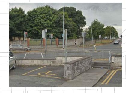
OFF STREET ACCESSIBLE CAR PARKING SPACE. A COMFORTABLE ACCESS FROM THE PARKING TO THE FOOTPATH SHOULD BE IMPLEMENTED. A RAMP COULD BE WITH THE STAIR. TACTILE PAVING FOR WARNING TO BE INCORPORATE IN THE START /END OF THE EXTERNAL STAIRS. DIMENSIONS OF 2400x4800 FOR THE ACCESSIBLE PARKING BAY AND A 1200 MM CLEAR ACCESS ZONE TO BOTH SIDES AN D THE END OF SPACE.
