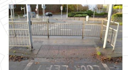
CHECK CROSSFALL IN STAGGERED CROSSING POINT: LEAVES, ACCUMULATED WATER AND SLIPPERY GROUND CAN RESULT A HAZARD. DRAINAGE SYSTEM SHOULD BE REVISED. THIS TYPE OF CROSSING SHOULD HAVE ALSO TO BE REVIEWED. A CENTRAL REFUGE ISLAND IN ONE STAGE WITH PROPER RED BLISTER TACTILE PAVING SHOULD BE RECOMMENDED TO AVOID PEOPLE TO GET STUCK BECAUSE OF THE NARROW WIDTH.
