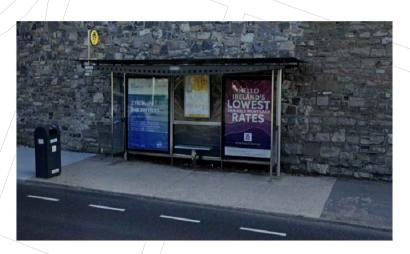
BUS STOP. A KASSEL KERB SHOULD BE INCORPORATED AND TEXTURED SURFACE TO WARN PEOPLE WITH VISUAL IMPAIRMENTS. AN ADEQUATE UPSTAND HEIGHT (180 MM) SHOULD BE ENSURED TO ADAPT FOR A KNEELING SUSPENSION OF LOW-FLOOR BUSES.
