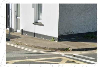
UNCONTROLLED CROSSING POINT. BUFF OR GREY" TACTILE P SHOULD BE CONSIDERED DEPTH OF 1.2 M, GRADIENT 1:12 MAX LEVEL DIFFERENCE OF DISHED KERB: 6MM
