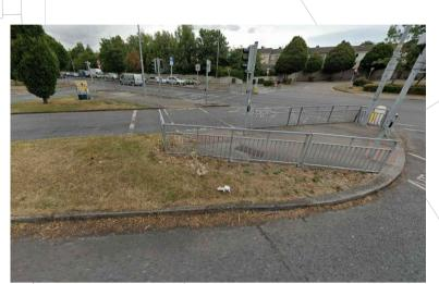
THE MULTI-STAGED CONTROLLED CROSSING POINT IS REDUCED IN THE DESIGN PROPOSED TO ONE ONLY STAGE. THIS SHOULD AVOID THE CONFUSION FOR MULTIPLE AUDIBLE SIGNALS. RED BLISTER TACTILE PAVINGS SHOULD BE PROVIDED IN THE NEW CENTRAL REFUGE ISLAND.
