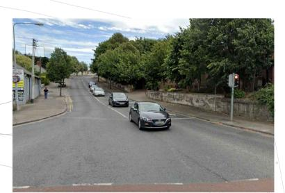
A CONTROLLED CROSSING POINT IS PROPOSED IN THE PROJECT DESIGN. MEASURES OF ACCESIBILITY FOR THIS TYPE OF CROSSING SHOULD BE IMPLEMENTED. RED BLISTER TACTILE PAVING. DISHED KERBS. A FULL WIDTH OF DROPPED KERB WITH A MIINIMUM OF 2400 MM WIDE AND 800 MM (2 SLABS) DEEP. THE 'DIMPLES' IN THE TACTILE PAVING UNITS SHOULD BE ALIGNED AND TOP OF THE DROPPED KERB SHOULD BE PAINTED IN WHITE
